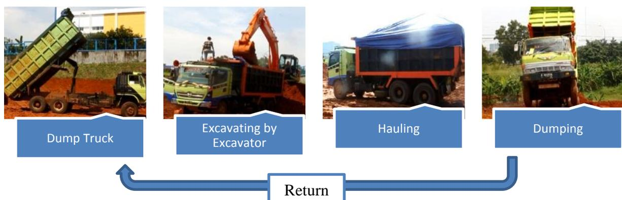
Gambar 2.5 Proses Hauling and Earthmoving
