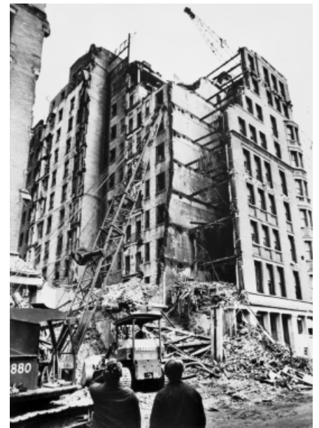
Fig. 3. Gladstone Hotel, Philadelphia, during demolition in 1971, showing steel beams spanning between exterior and interior bearing walls. Courtesy of the Library of Congress, Prints and Photographs Division, HABS PA, 51-PHILA, 425-1.
