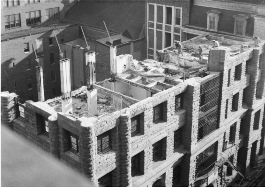
Fig. 4. American Life Building, Philadelphia, during demolition in 1961, showing cast-iron columns (below arrows) in the interior at left and exterior bearing walls. Courtesy of the Library of Congress, Prints and Photographs Division, HABS PA, 51-PHILA, 257-7.
