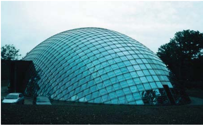
▲ 8.30 Seed House and Forestry Centre, Marche-en-Femenne, Belgium, Samyn et Associés, 1996. Exterior view.
