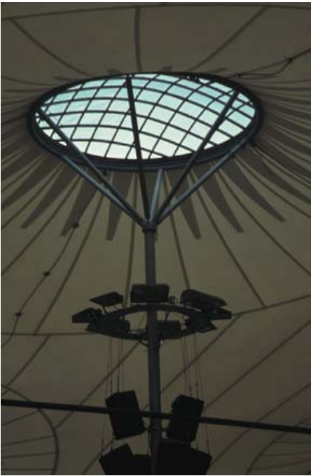
▲ 8.1 Stellingen Ice Skating Rink and Velodrome, Hamburg, Germany, Silcher, Werner + Partners, 1996. Daylight enters the junction between the flying-strut and the fabric membrane.
