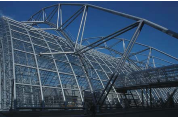
▲ 8.13 Trade Fair Glass Hall, Leipzig, Germany, Ian Ritchie Architects, 1996. Exterior trusses support the vaulted grid-shell.
