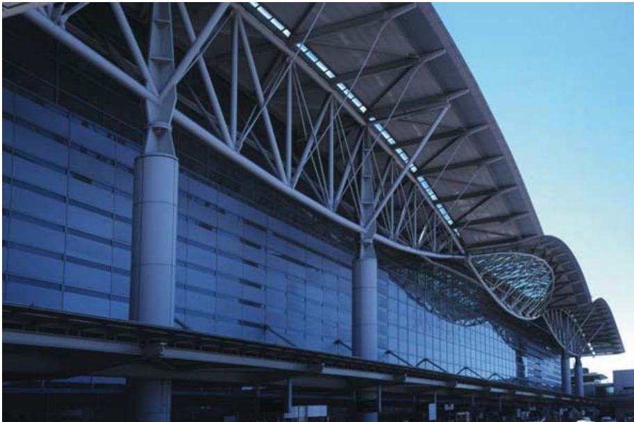
▲ 8.2 San Francisco International Airport, USA, Skidmore Owings & Merrill LLP, 2000. A two-dimensional truss transforms into three dimensions over the central span of the terminal.
