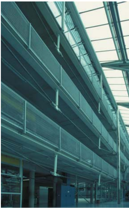
▲ 8.17 School at Waidhausenstraße, Vienna, Austria, Helmut Richter, 1995. Composite steel walkway beams.
