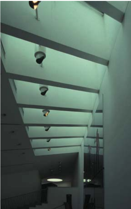
▲ 8.32 Mönchengladbach Museum, Germany, Hans Hollein, 1982. Beams screen and reflect light into the gallery below.
