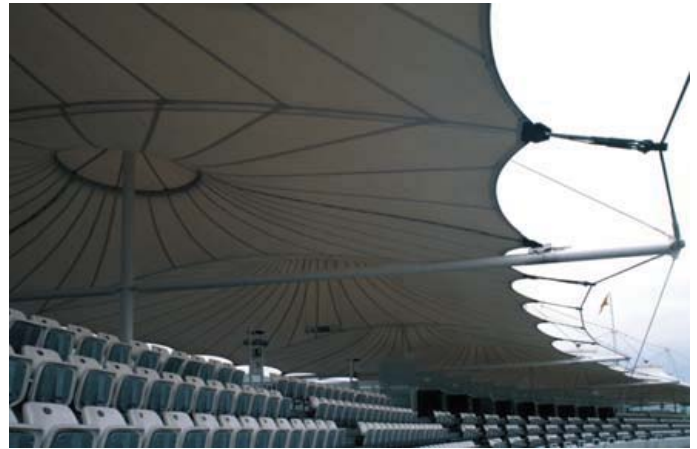
▲ 8.35 Mound Stand, Lord's Cricket Ground, London, England, Michael Hopkins and Partners, 1987. Underside of the fabric roof.
