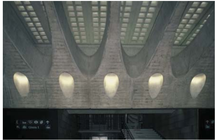
▲ 8.12 Stadelhofen Railway Station, Zürich, Switzerland, Santiago Calatrava, 1990. Integration of structure and artificial lighting.
