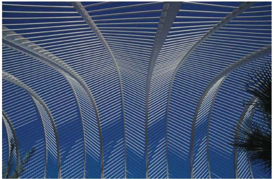
▲ 8.29 Shade-structure arches and ribs.
