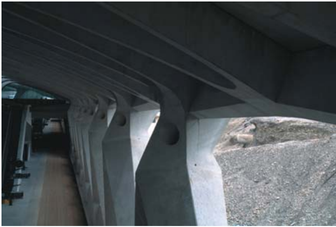
▲ 8.11 Recessed lights in stub columns.
