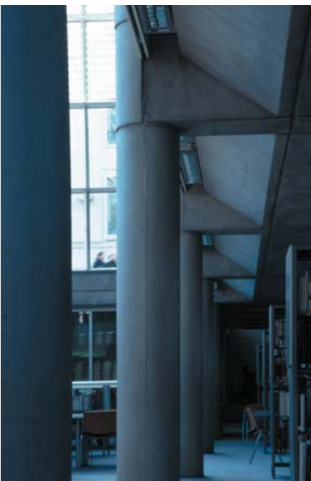
▲ 8.20 Bevelled and set-back beams.
