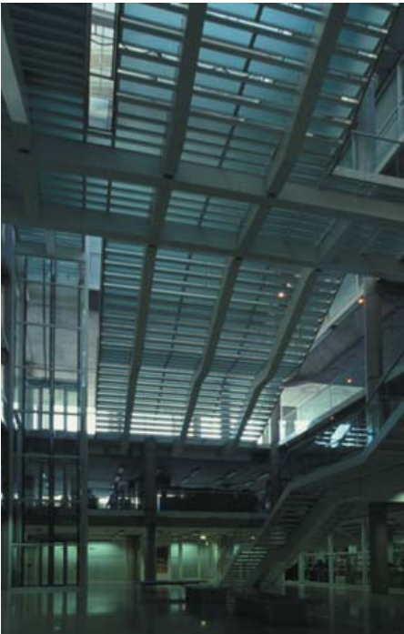
▲ 8.19 Carré d'Art, Nîmes, France, Sir Norman Foster and Partners, 1993. Glass stair-treads and the supporting structure in the atrium.
