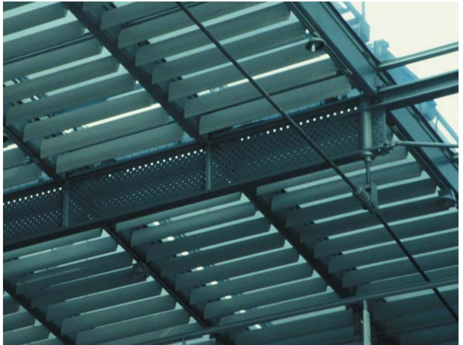
▲ 8.21 Schools of Geography and Engineering, Marne-la-Vallée, Paris, France, Chaix & Morel, 1996. A finely perforated web of a steel beam.
