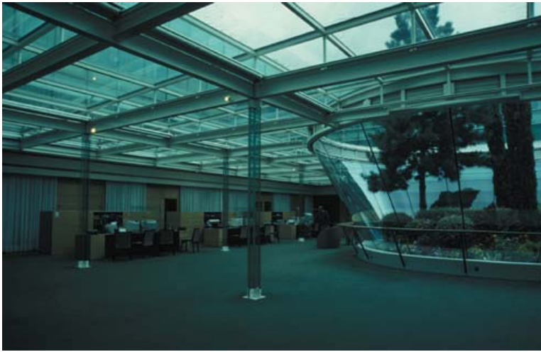
▲ 8.24 Town Administrative Centre, Saint-Germain-en-Laye, Paris, France, Brunet and Saunier, 1995. Glass columns support roof beams.
