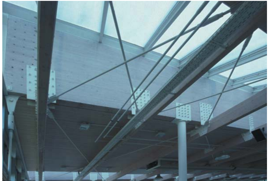
▲ 8.33 Business School, Öhringen, Germany, Günter Behnisch & Partner, 1993. A primary beam with the skylight above and the roof below.
