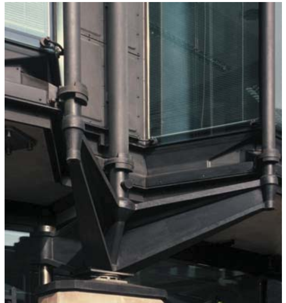
▲ 4.41 Metal columns, a cantilever bracket and a stainless steel rod behind a stone pier.
