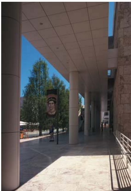
▲ 4.17 A colonnade supporting an elevated walkway alongside an external wall.
