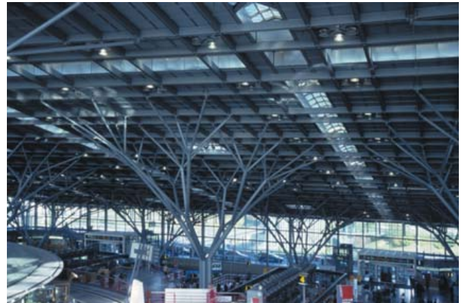
▲ 3.43 Stuttgart Airport Terminal, Germany, von Gerkan • Marg + Partner, 1991. Structural 'trees'.
