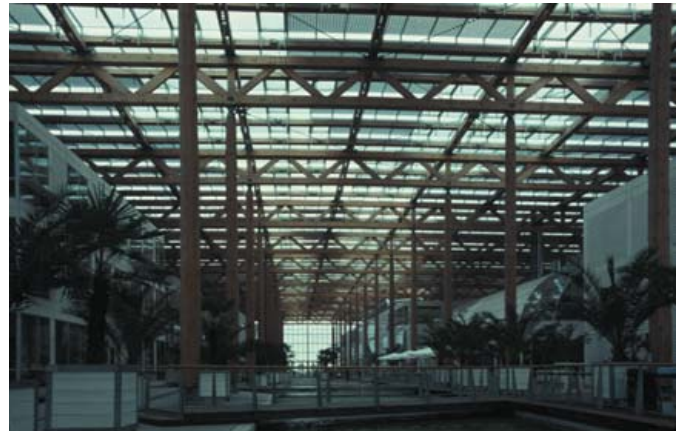
▲ 3.27 Interior timber structure.
