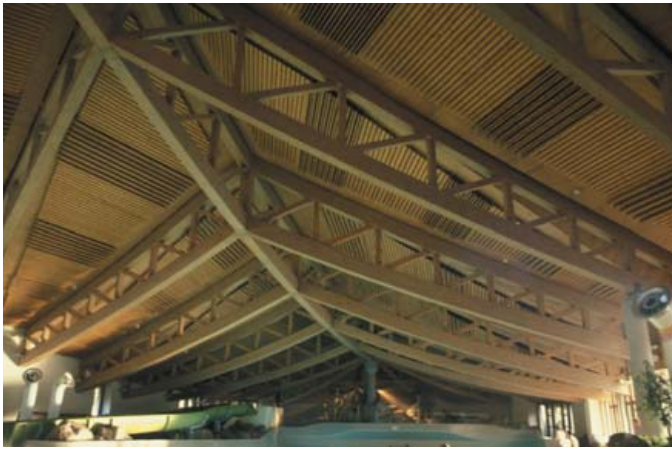
▲ 3.35 Roof structure over main pool.
