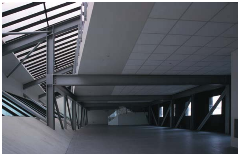
▲ 3.54 An interior office space where the sloping wall angles across the line of the truss.
