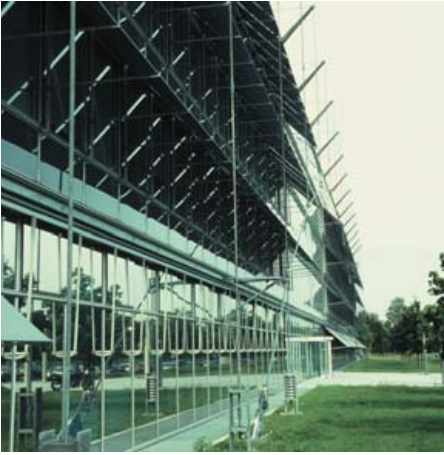
▲ 3.52 Exterior tension rods and springs.
