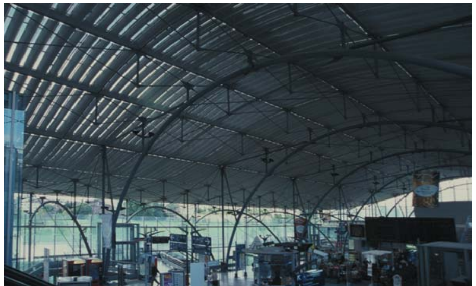
▲ 3.46 Unexpected interior arches in the TGV Station.
