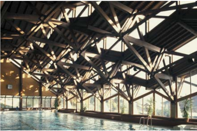
▲ 3.39 Visually complex roof structure over the pool.
