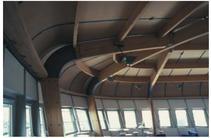
▲ 3.29 The curved roof structure.
