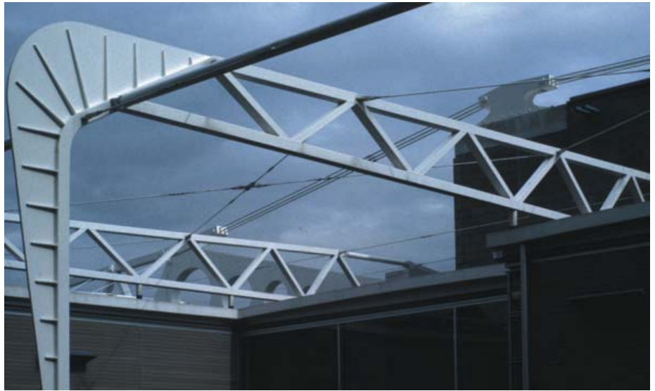
▲ 2.6 Innovatively detailed portal frame columns, with the core and an 'anvil' support for the trusses in the background.
