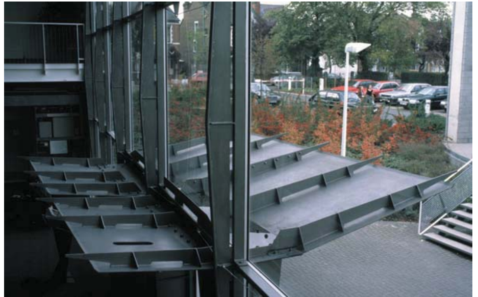
▲ 2.9 Refined structural detailing in the atrium and to the main entrance canopy.
