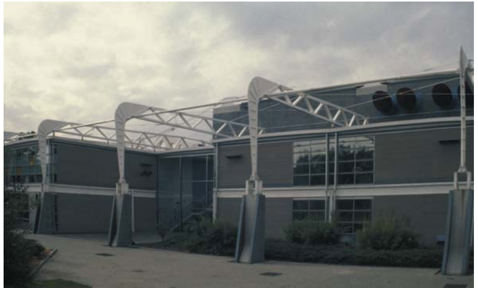
▲ 2.1 BRIT School, Croydon, London, England, Cassidy Taggart Partnership, 1991. Exoskeleton with the core behind the two-storey podium. Ventilation ducts protrude from the core wall.
