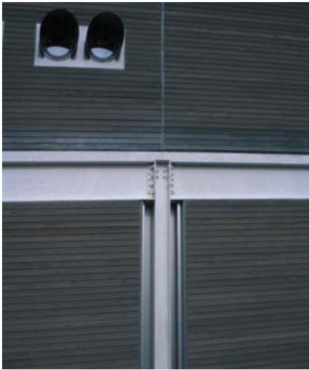
▲ 2.5 Exterior column recessed within an external wall.
