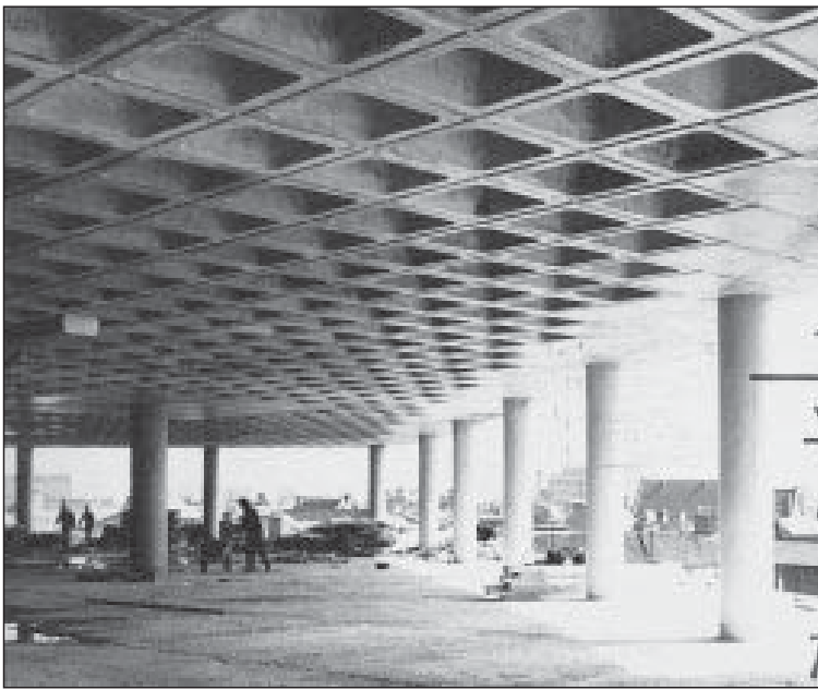
Fig. 5.19 Willis, Faber and Dumas office, Ipswich, UK, 1974; Foster Associates, architects; Anthony Hunt Associates, structural engineers. The coffered floor slab is a flat-slab structure with an 'improved' cross-section. (Photo: Pat Hunt)
