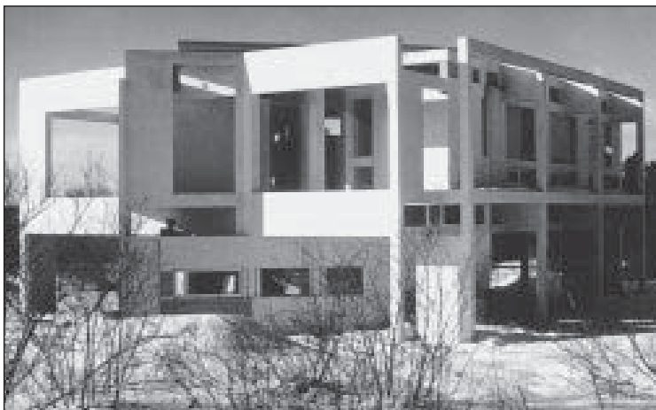
Fig. 5.18 Miller House, Connecticut, USA, 1970; Peter Eisenman, architect. Eisenman is one of a number of American architects, including Richard Meier (see Fig. 1.9), who have exploited the opportunities made possible by the continuous framework. This type of geometry, with its intersecting grids and contrasts of solid and void is only possible with a continuous structure.
