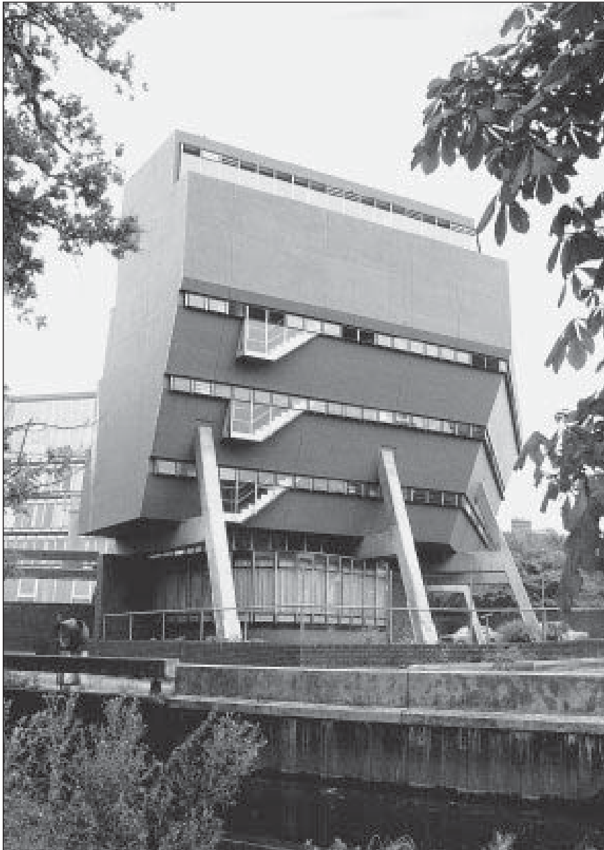
Fig. 5.17 Florey Building, Oxford, UK, 1971; James Stirling, architect. The Florey Building, with its crescent-shaped plan, complex cross-section and glazed wall, illustrates how the geometric freedom made possible by a continuous frame of in situ concrete can be exploited. (Photo: P. Macdonald)
