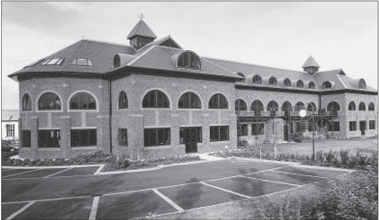
Fig. 5.6 Corinthian Court, Abingdon, UK; the Baron Willmore Partnership, architects; Glanville and Associates, structural engineers. The vertical structure of this three-storey office building, which measures 55 m by 20 m on plan and has few internal walls, is of loadbearing masonry. The floors are of reinforced concrete.
