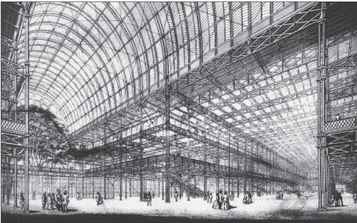
Fig. 7.25 Crystal Palace, London, UK, 1851; Joseph Paxton, architect/engineer. The Crystal Palace was a truly high-tech building and an inspiration to generations of modern architects. Unlike many twentieth-century buildings to which the label High Tech has been applied, it was at the forefront of what was technically possible at the time. The major decisions affecting the form of the building were taken for technical reasons and were not compromised for visual or stylistic effect. The building has technical shortcomings, such as the poor durability of the many joints in the external skin, but in the context of a temporary building it was appropriate that these were given a low priority.
