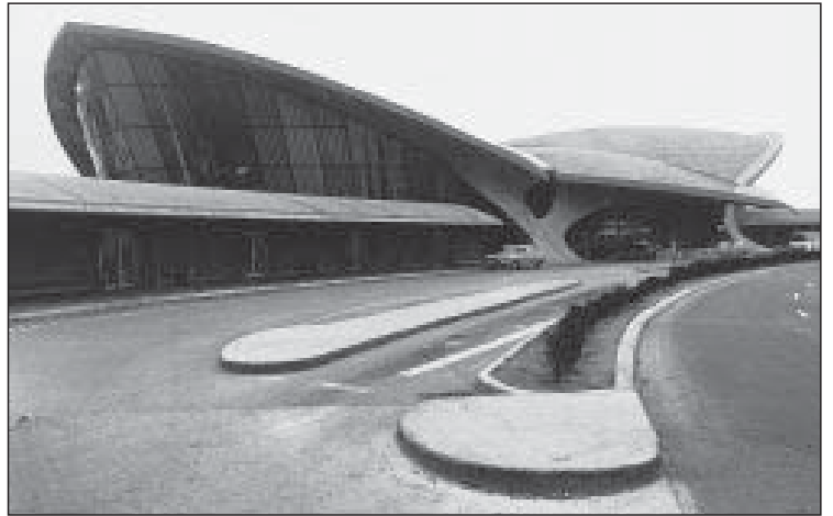
Fig. 7.45 TWA Terminal, Idlewild (now Kennedy) Airport, New York, USA, 1962; Eero Saarinen, architect; Amman and Whitney, structural engineers. The form here was far from ideal structurally and strengthening ribs of great thickness were required at locations of high internal force. The structure was therefore inefficient but construction was possible due to the relatively modest spans involved. (Photo: R. J. Mainstone)
