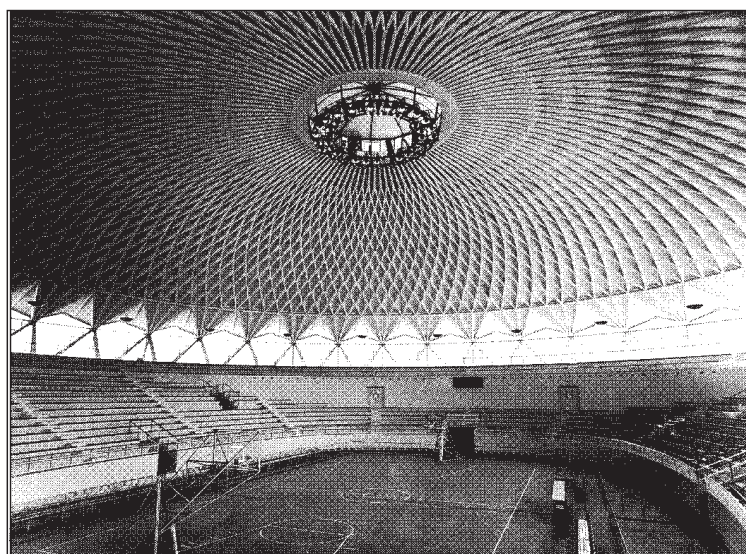
Fig. 7.15 Palazzetto dello Sport, Rome, Italy, 1960; Pier Luigi Nervi, architect/engineer. This is another example of a building with a form determined solely from structural requirements. The compressive form-active dome is a composite of in situ and pre-cast reinforced concrete and has an 'improved' corrugated cross-section. (Photo: British Cement Association)
