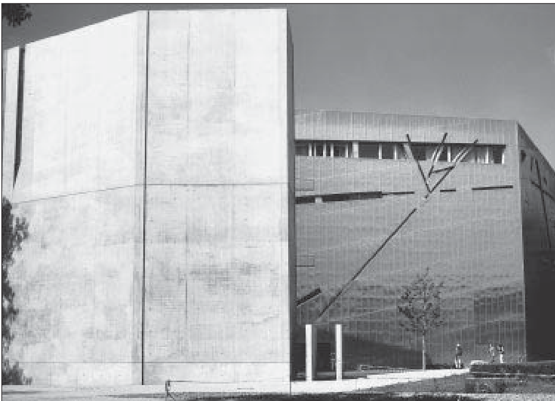
Fig. 7.42 Jewish Museum, Berlin, 1999; Daniel Libeskind Architecturburo, architects. The use of a reinforced concrete structural framework has allowed both a highly sculptured overall form to be created and a high degree of freedom to be achieved in the treatment of the non-structural cladding of the exterior.
