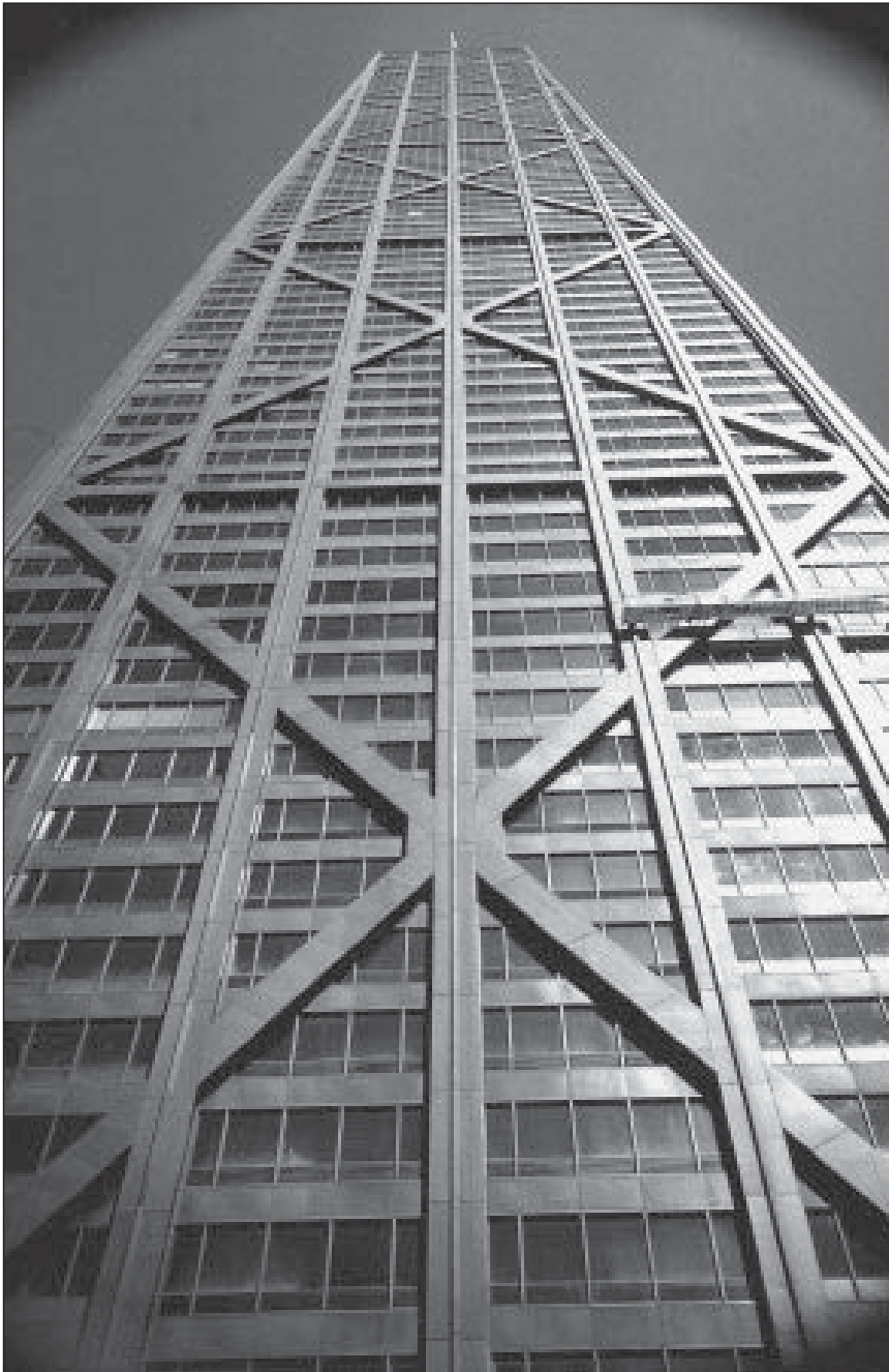
Fig. 7.21 John Hancock Building, Chicago, USA, 1969; Skidmore, Owings and Merrill, architects and structural engineers. The trussed-tube structure here forms a major component of the visual vocabulary. (Photo: Chris Smallwood)
