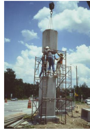
ERECTION OF PRECAST CONCRETE PIERS AND GIRDERS
