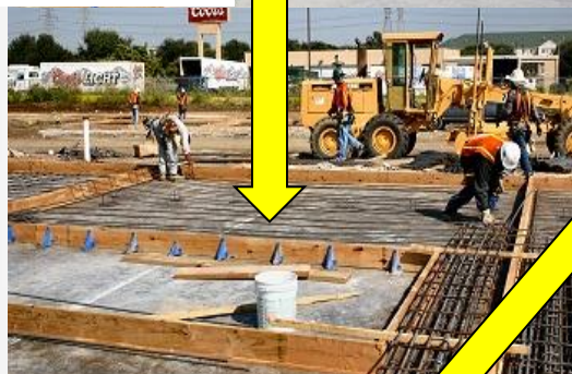
form-work (flat slab)
