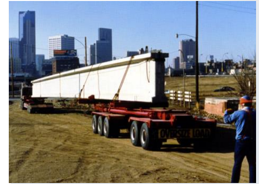
TRANSPORTATION OF PRECAST CONCRETE ELEMENTS
