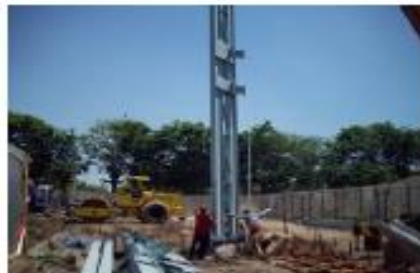
Column erection P2 C1
