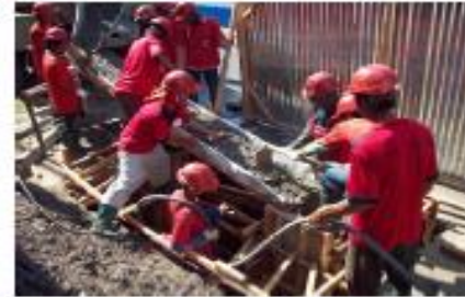
Pouring concrete for pipe rack column
