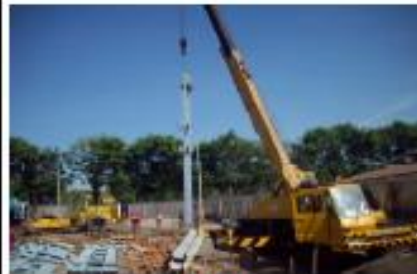
Column erection C1
