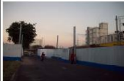
Column erection P1 & P2
