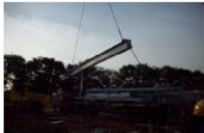
Unloading steel material
