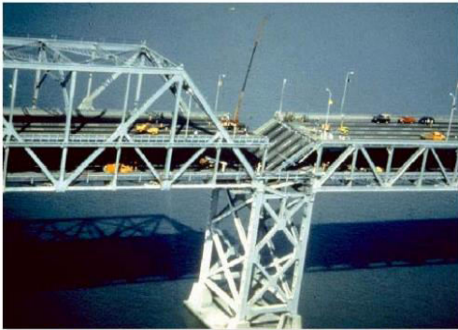
1989 Earthquake in Loma Prieta, California Oakland Bay Bridge failure.
