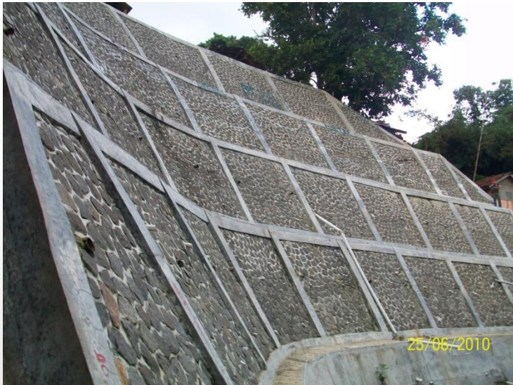
Dinding penahan tanah
