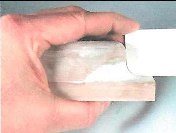
Step D Quick-drying polyfilla is used for final finishing. The DryDex® brand of polyfilla contains a colourant so that it starts pink and hardens to a white colour.
