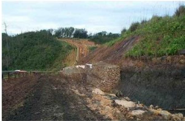
(Retaining wall Gabion)
